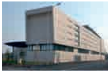
3. Departmental Archives of Yvelines, rear façade: the stores (Architects: Bernard Feypell and associates). Photo DA Yvelines.
