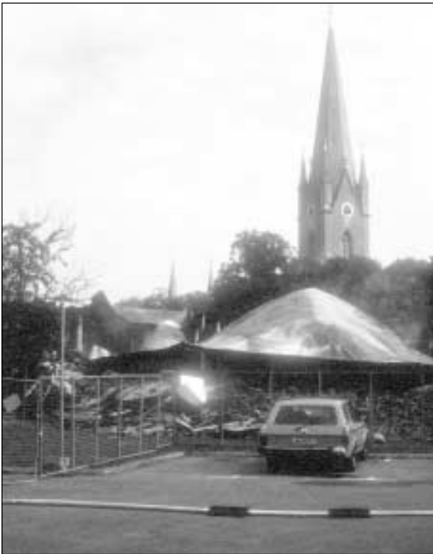
The library after the fire
